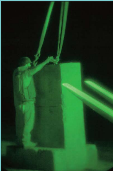
Above: Kellogg Brown and Root personnel hook a crane to an Alaska barrier so it can lift the heavy cement and maneuver it into place at a traffic control point (TCP) June 8.
